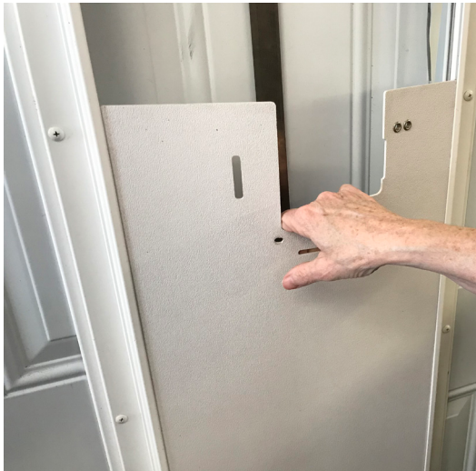
Pull Upper Cover out of frame
