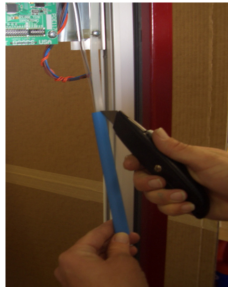
Cut blue sleeve lengthwise.
